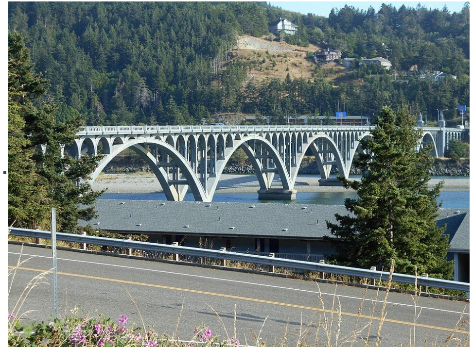
Bridge across the Rogue River in Gold Beach, OR
